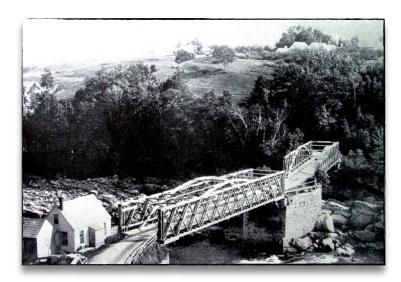
Lisbon Falls to Durham Androscoggin River Toll Bridge, c.1890. This bridge was replaced in 1895. The iron arches are later additions to the original wood construction.
