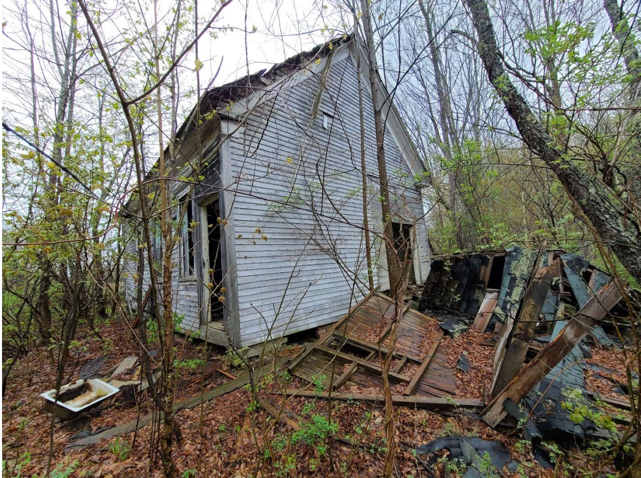
View of the back of the building
