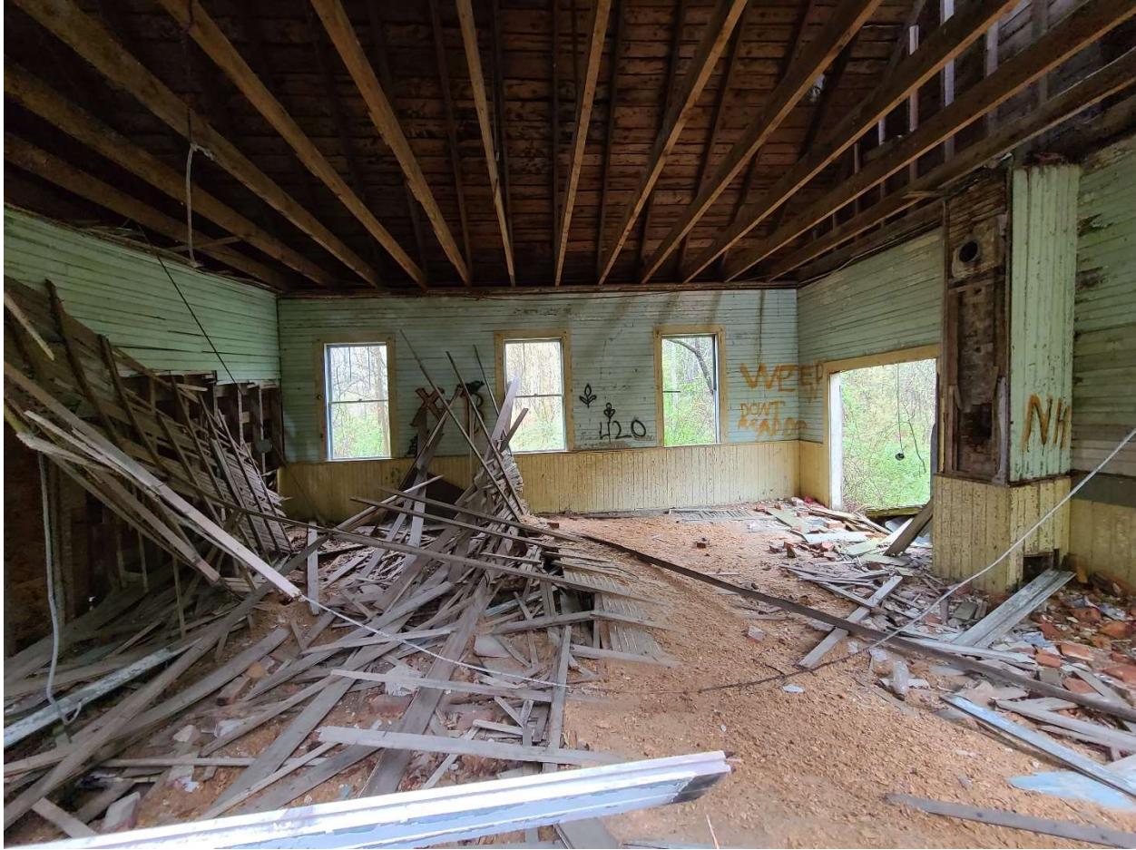
View of the inside of the building
